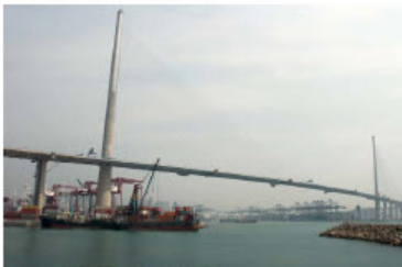
Figure 1: General view of Stonecutters Bridge
