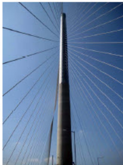
Figure 2: Mono tower and stay cables
